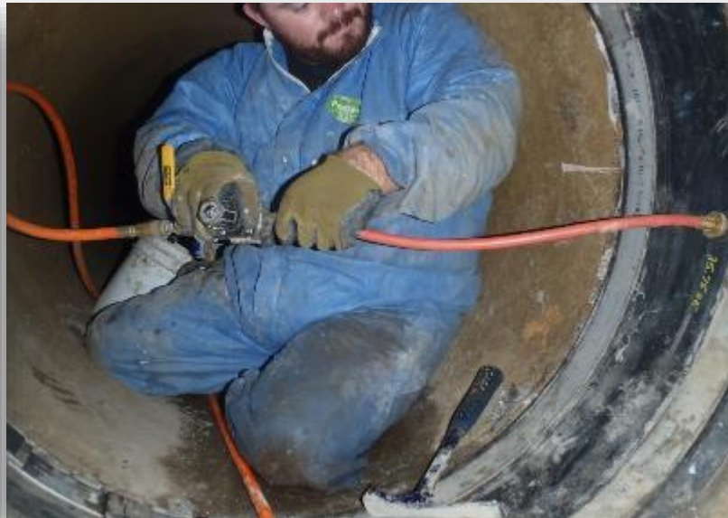
Test seals for leakage
