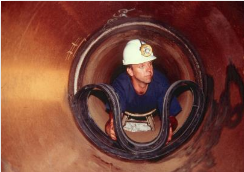
Prepare joint and install seals
