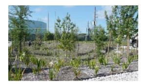
Detention is built to mitigate the effects or impact of increased impervious cover (development) on the existing drainage system. Stormwater detention volume is based on increased impervious surfaces and correspondingly, adjustments to impervious surface area are based on the volume of detention of provided. The IDM details how to size the outlet or discharge pipe. Detention requires routine inspection and maintenance typically involves removal of silt build-up in the basin and at the outfall.
