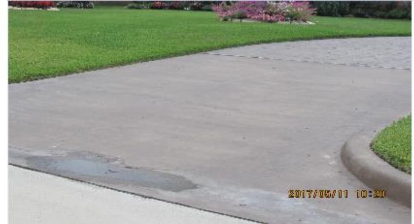
**Option 2:** Grade the subgrade to proper slope and form the driveway to meet the new grades /slope. You would see the finished dirt with the proper slope. Homeowner will finish the driveway with their desired finish at their cost. (Driveway must be finished 2 weeks after it's been prepped by the City.)
