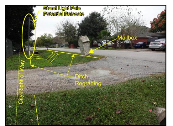
MAILBOX REPLACEMENT/PROTECTION AND STREET LIGHT REPLACEMENT/PROTECTION • Current Design: Protect mailbox structures and street light poles in place • Alternate Design: Replace mailbox structures with standard mailbox and street light poles; protect remaining in place • Additional Cost: ≈ \$230,000
